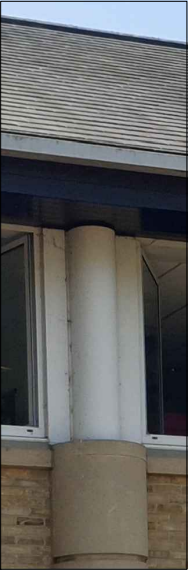
ALUMINIUM POWDER COATED FINISH TO MATCH EXISTING COLUMN
