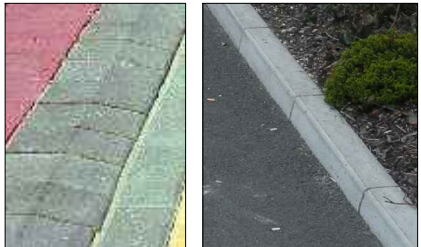
PCC Half battered Kerb 125x255mm
