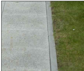
PCC Pin Kerb 150x50x915mm
