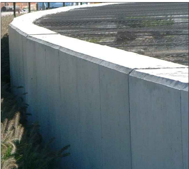
Fairfaced concrete retaining walls
