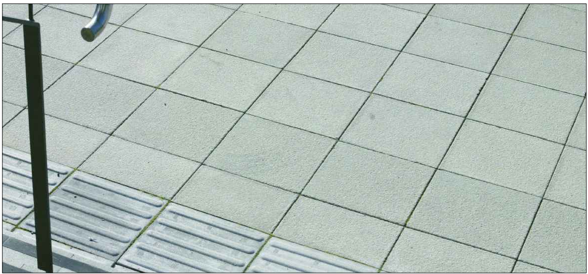
Paving slabs to pedestrian walkways, 450x450mm Marshalls Saxon textured to match existing / Natural or equivalent approved
