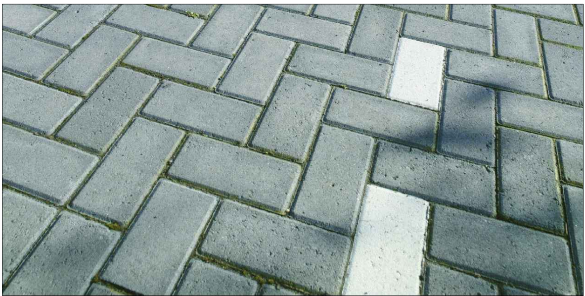
Marshalls Keyblock, 200x100mm - Charcoal or equivalent approved - Herringbone pattern
