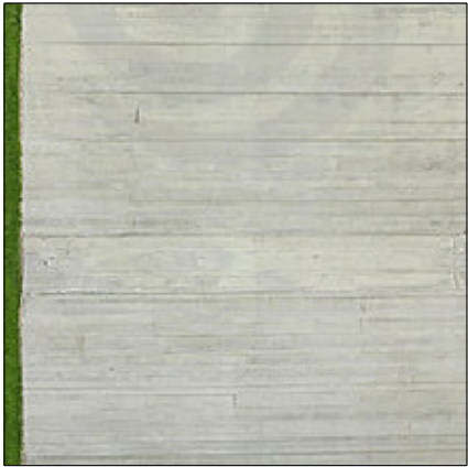
CONCRETE Location: Plinth detail and feature entrance portico.
