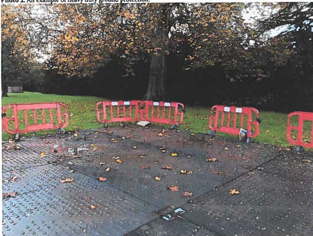
Photo 2. An example of heavy duty ground protection.
