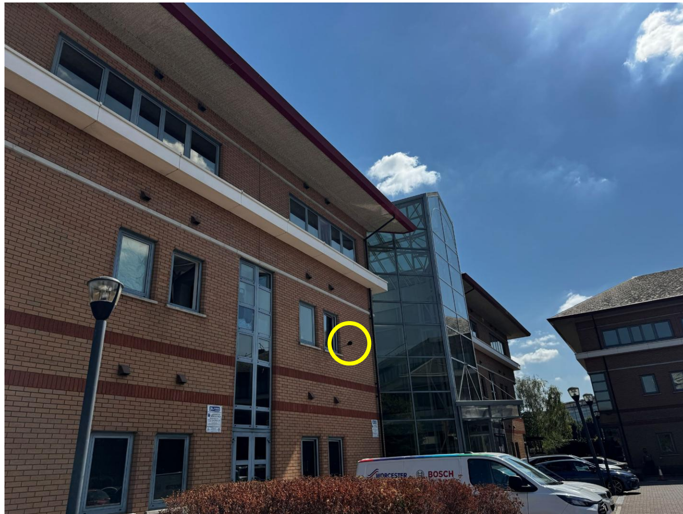
FIGURE 2: UNATTENDED MONITORING POSITION (NMP1) – LOOKING EAST TOWARDS FRONT SOUTHWEST ENTRANCE FAÇADE OF MONDIAL HOUSE
