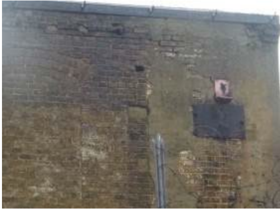
Photograph 10. Superficial cracks in single-skin brickwork of B2 (western elevation).
