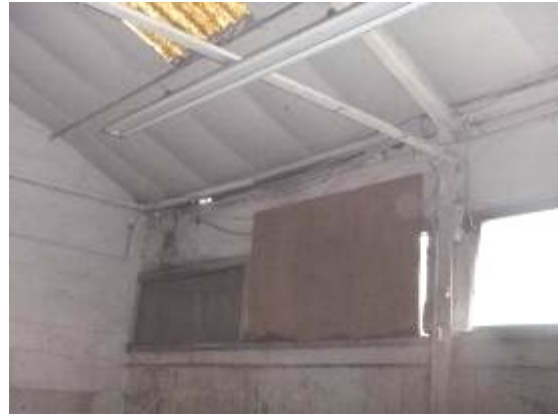
Photograph 6. Daylight visible at the eaves on the southern side of B1.
