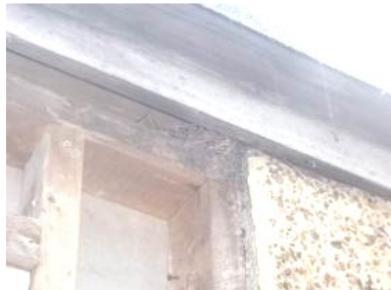
Photograph 13. Bird nesting material present in gap under fascia (northern elevation).
