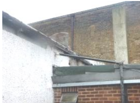
Photograph 4. Missing section of fascia along eaves of B1 (southern elevation).
