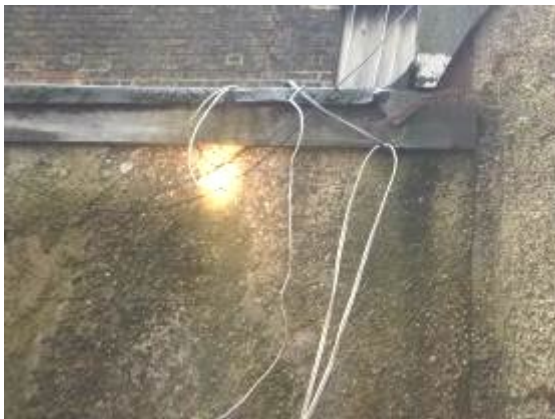
Photograph 12. Tight timber fascia to wall on single storey extension (northern elevation).
