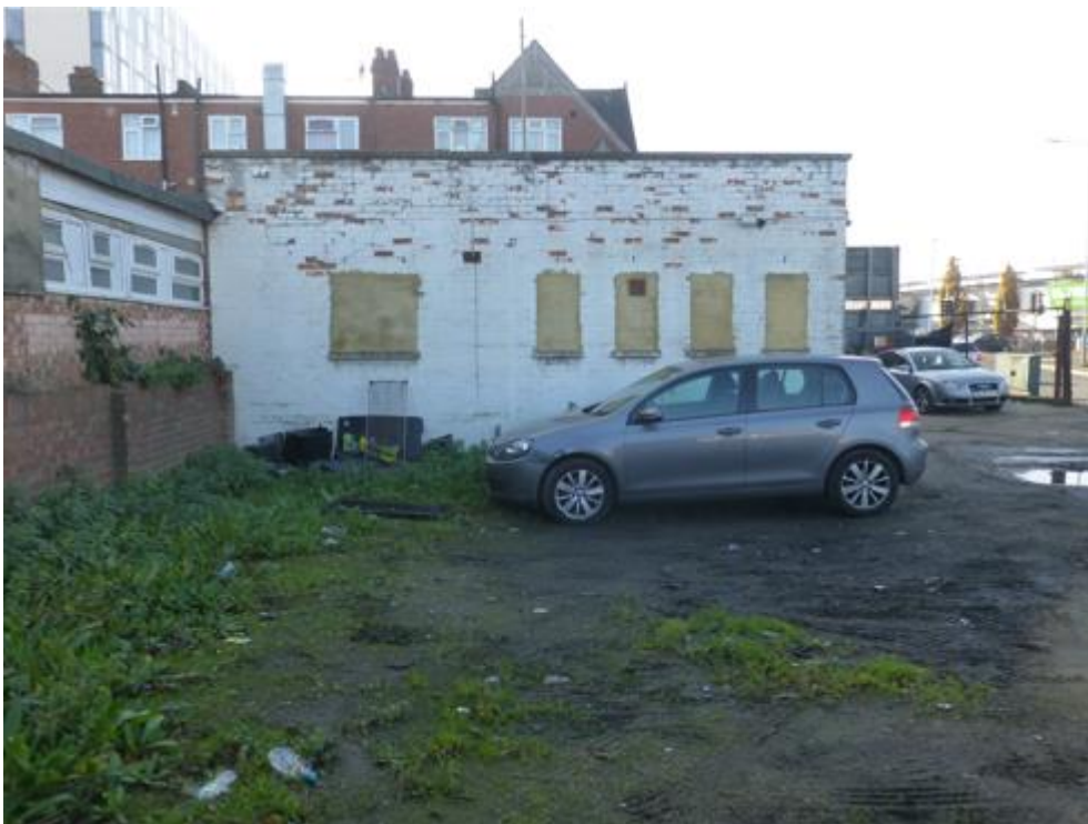
Photograph 8: View to rear of shop extension
