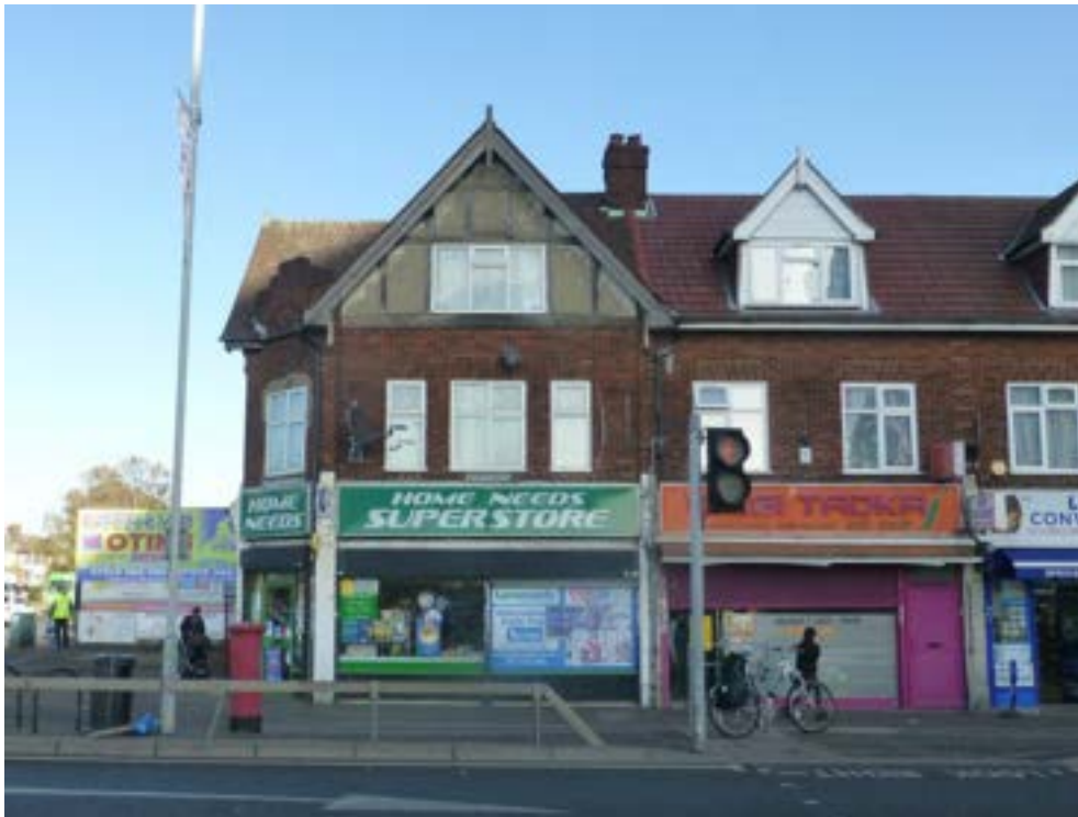
Photograph 2: View to front of 152-154 Uxbridge Road
