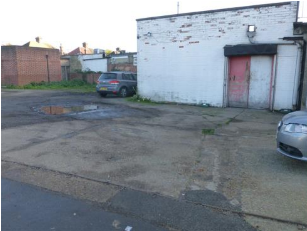
Photograph 7: View of shop service entrance and yard area
