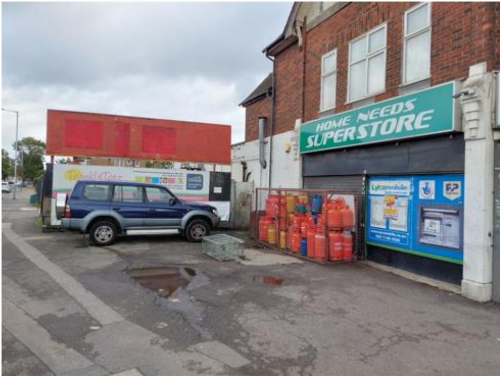
Photograph 3: View of side of property showing gas cylinder storage
