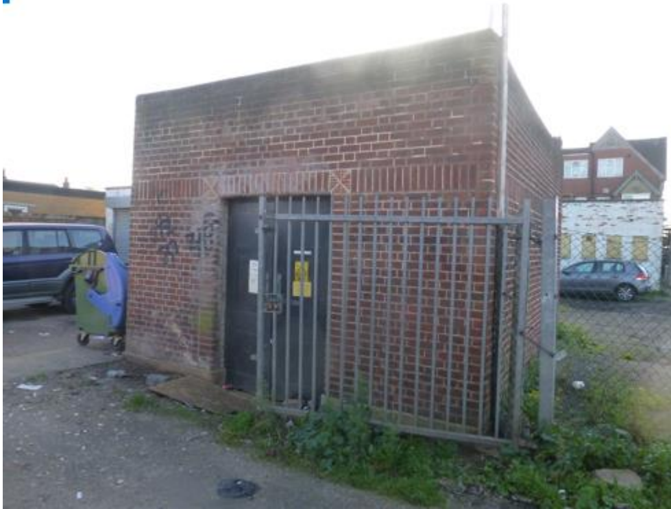
Photograph 9 : View of electricity substation showing enclosed brick structure
