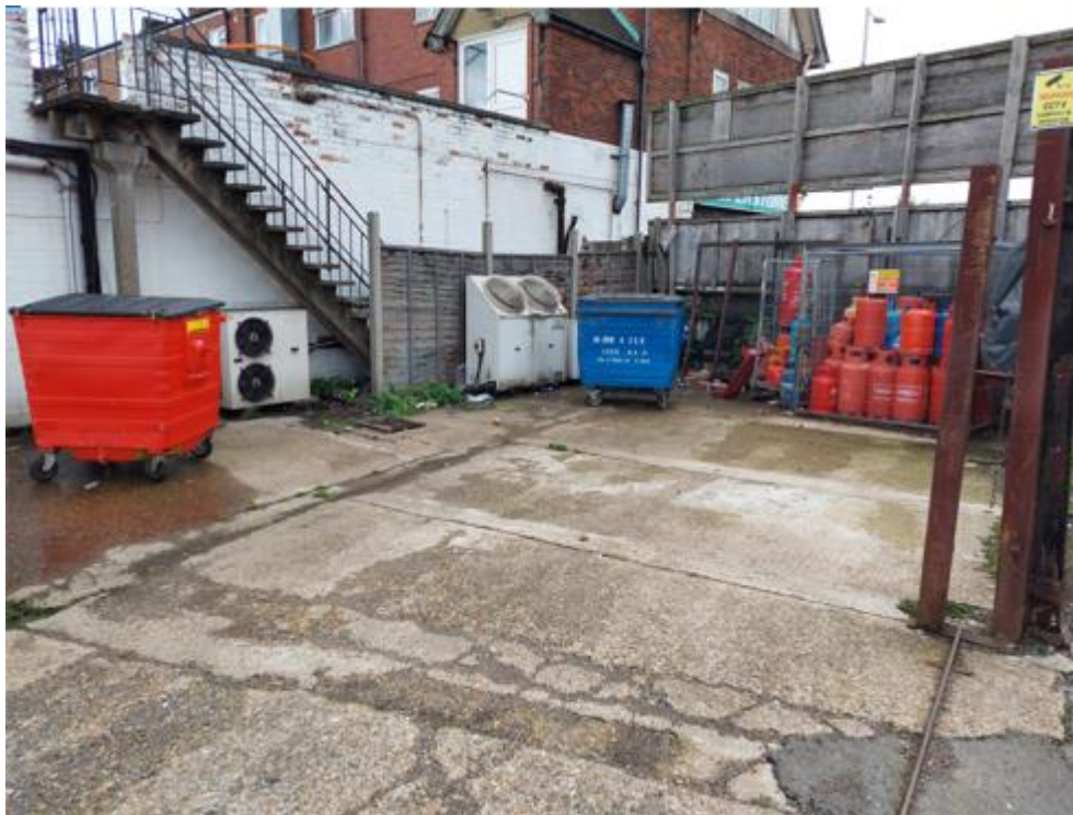
Photograph 4: View of access area to rear of advertising hoarding
