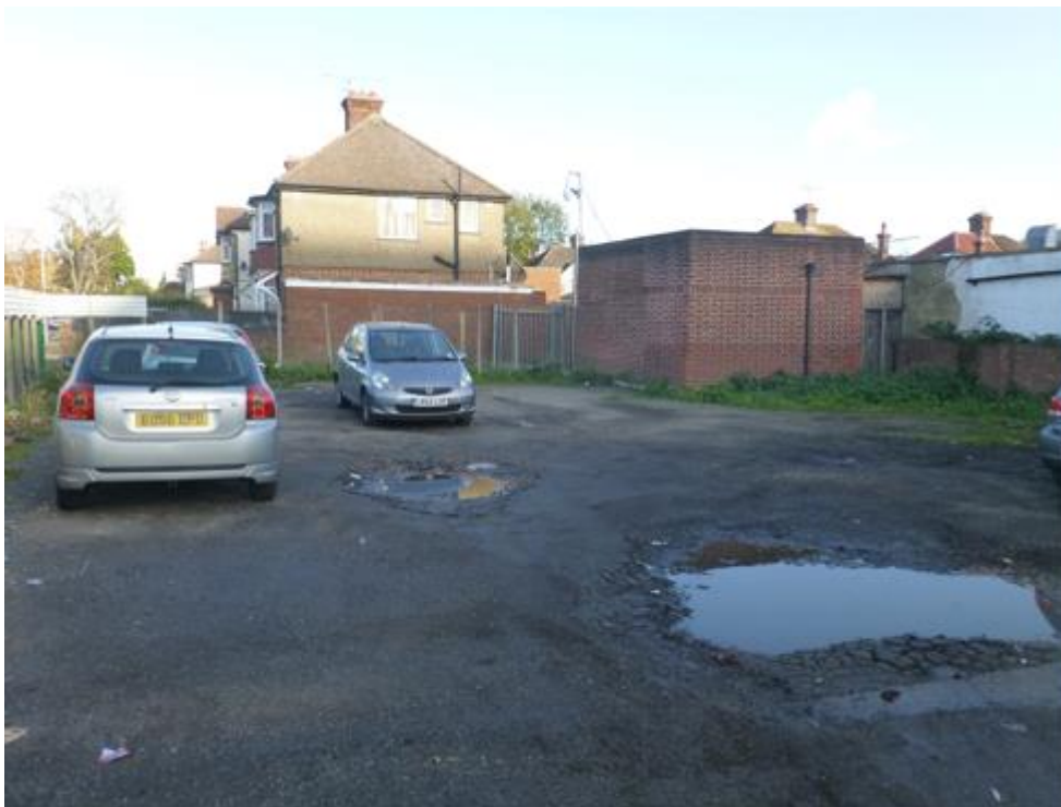
Photograph 6: View of rear yard area showing electricity substation
