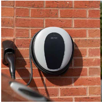
Wall mounted domestic electric charger 7kw mode 3
