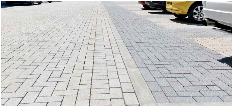
Permeable Block Paving: Marshalls or Tobermore or similar equivalent; colour TBC; installed in accordance with the manufacturer's instructions
