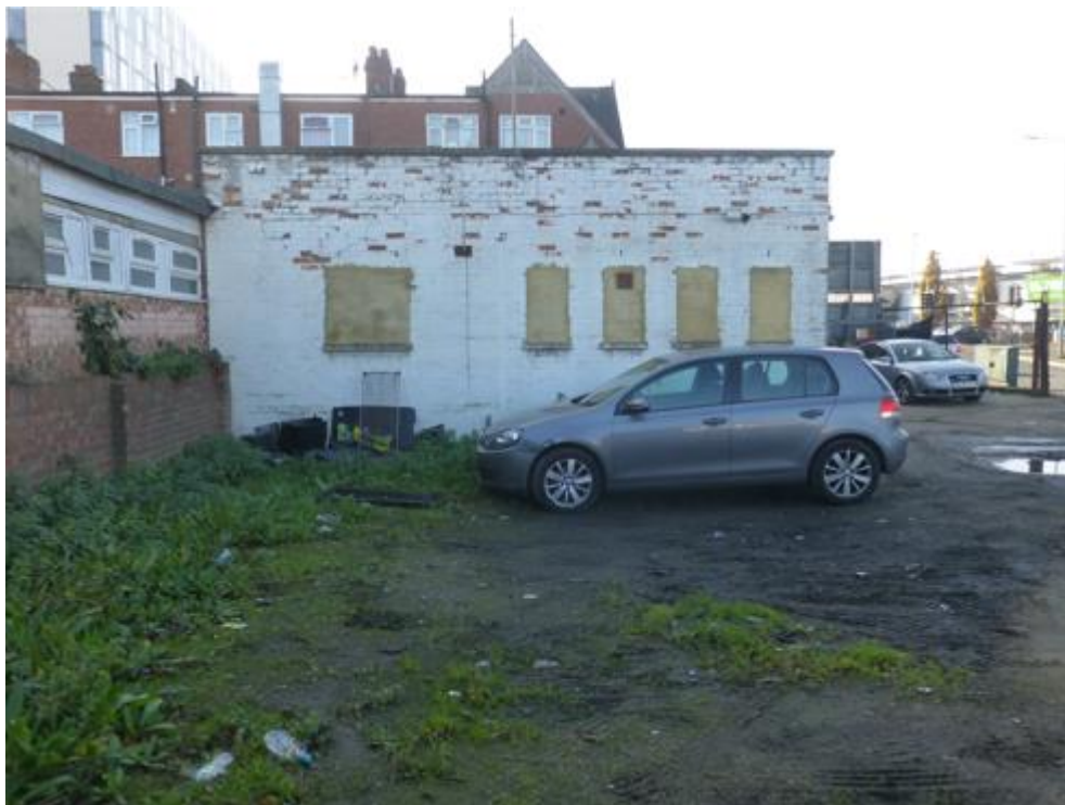
Photograph 8: View to rear of shop extension
