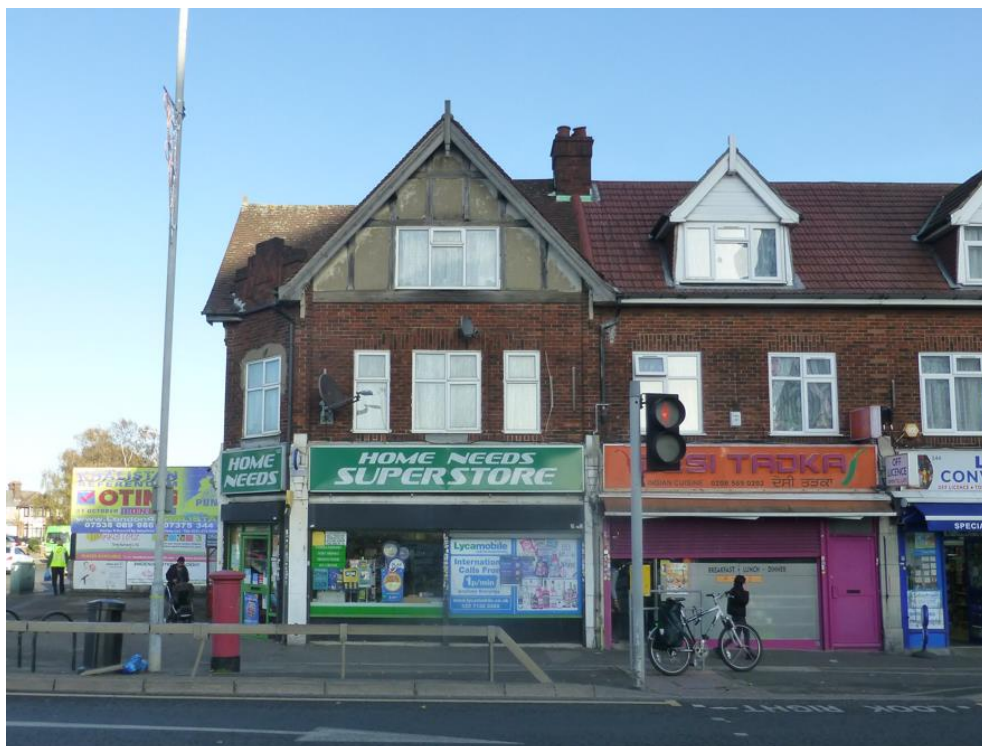
Photograph 2: View to front of 152-154 Uxbridge Road
