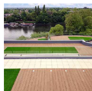
Timber Decking & Paving Tiles
