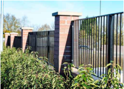
Vertical Flat Bar Railings: Colour: Black; 1200mm high (circa)
