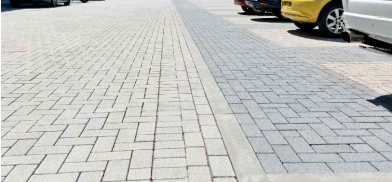
Permeable Block Paving: Marshalls or Tobermore or similar equivalent; colour: TBC; installed in accordance with the manufacturer's instructions
