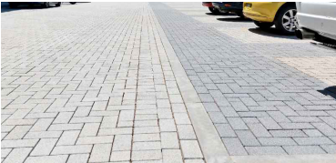
Permeable Block Paving: Marshalls or Tobemore or similar equivalent; colour TBC; installed in accordance with the manufacturer's instructions
