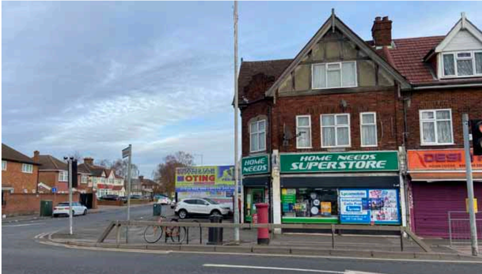
Photo 8: View from pedestrian crossing on Uxbridge Road looking north of existing building to be demolished.
