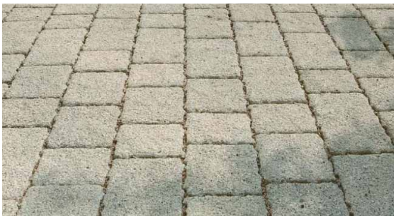
Permeable paving
