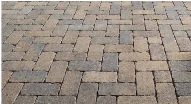
Permeable block paving
