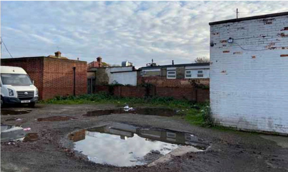
Photo 3: View from within the site looking north-east towards the existing substation and immediately adjacent single storey buildings.
