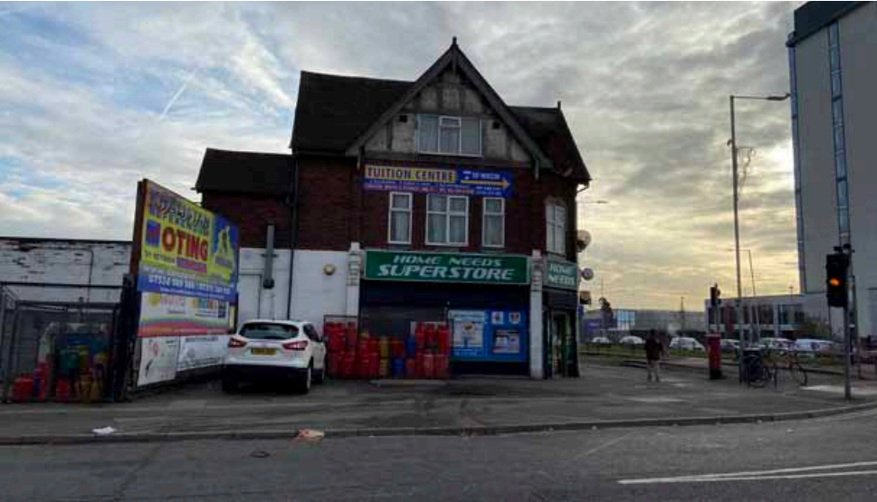
Photo 7: View of western elevation of existing building to be demolished from the road junction of Brookside Road and Uxbridge Road.
