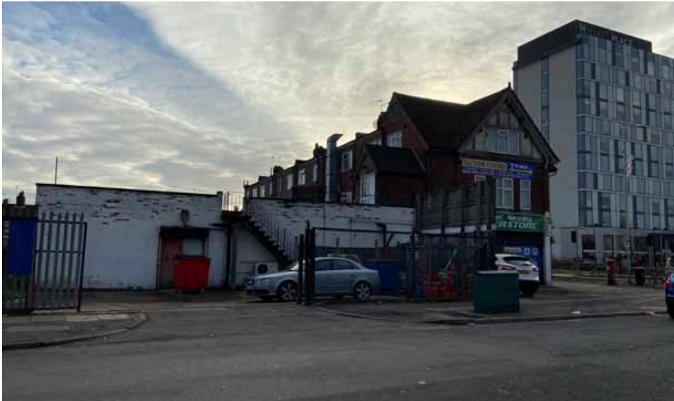
Photo 2: View looking south-east from Brookside Road towards southern part of application site.
