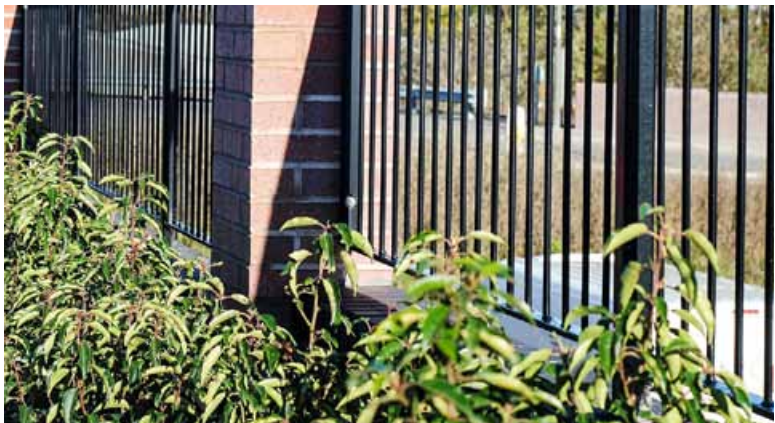
Road frontage to Plot 1: Metal railings and hedgerow planting
