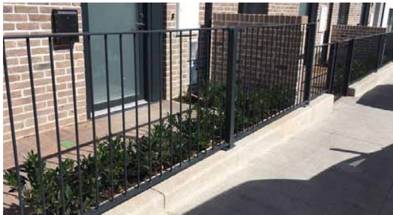
Flat top vertical bar metal railings along road frontage to Plot 1
