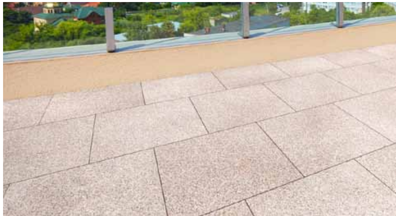
Roof Amenity Areas: Paving tiles on pedestals
