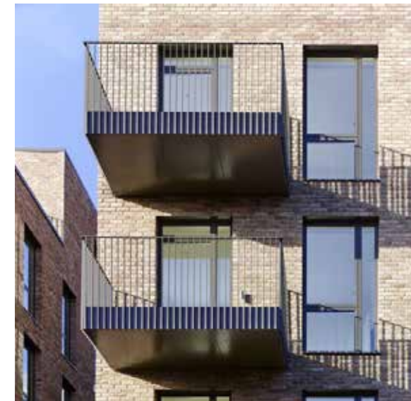
Contemporary steel balcony designed with flat bar balustrades projecting down over edge profile
