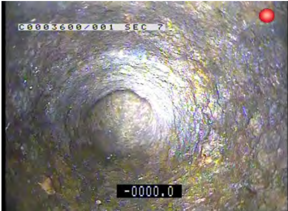
RWPX_c0b022f0-c988-4763-8b87-8dd4613abe74_20170824_132930_971.jpg, 00:00:00, 0.00m Start node type, manhole, reference number: SW2
