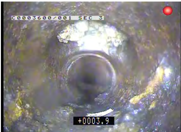
GULLYX_bff1f71b-96d5-4cfb-8bc6-4c75d21ddf41_20170824_130842_284.jpg, 00:01:17, 3.90m Junction at 12 o'clock, diameter: 100mm
