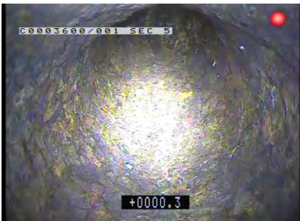
RWGX_f39017c3-8a31-43f6-8028-c3a3f333a637_20170824_1 31826_322.jpg, 00:04:16, 0.30m Finish node type, gully, reference number: RWG
