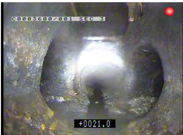
GULLYX_0033bda3-d509-497c-bbc3-1dc352e9ddb4_20170824_131253_547.jpg, 00:03:11, 21.00m Finish node type, manhole, reference number: GULLY
