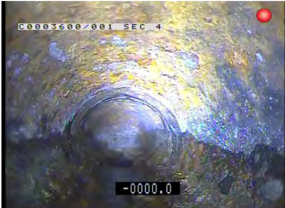
RWPX_d59d8097-ca9d-4a8f-a9d1-12efe58f5bc6_20170824_131513_067.jpg, 00:00:00, 0.00m Start node type, manhole, reference number: SW1
