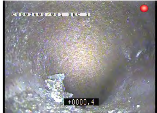
RWG1_f7727c03-b052-402c-98d4-87d5b4573e5b_20170824_125937_540.jpg, 00:00:29, 0.50m Survey abandoned / Unable To Traverse Camera Down
