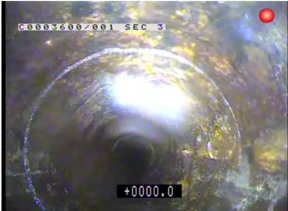
GULLYX_22c54bfb-4af5-41ef-abdb-1e6d672bafde_20170824_130748_949.jpg, 00:00:00, 0.00m Start node type, manhole, reference number: SW1
