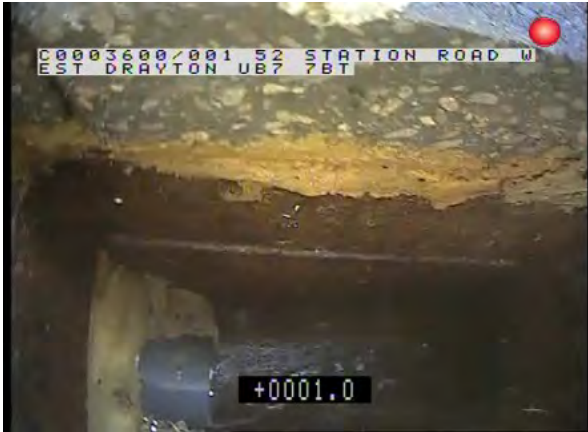
RWG1_69213870-0e87-463f-b282-60f6e9c5ee1f_20170824_125825_786.jpg, 00:00:00, -0.01m General photograph taken at this point / Overview
