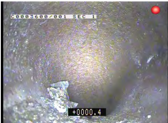
RWG1_b5b79b33-aecc-47b1-adaf-fec0bbae398e_20170824_125903_053.jpg, 00:00:29, 0.40m Line deviates down
