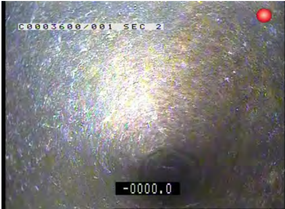
RWG2X_1baada2c-5331-42c1-bf49-12e2365e9bdc_20170824_130246_644.jpg, 00:00:00, 0.00m Start node type, gully, reference number: RWG2
