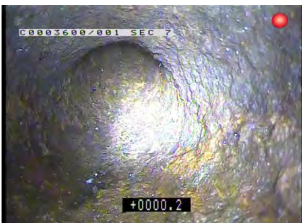
RWPX_fb4cb278-faa2-44d5-b9d4-a4d607830da4_20170824_132937_250.jpg, , 0.20m Line deviates up
