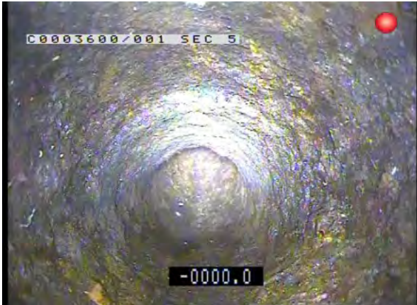
RWGX_35fcc129-c86f-4c07-9370-31b634003727_20170824_1 31729_547.jpg, 00:00:00, 0.00m Start node type, manhole, reference number: SW1
