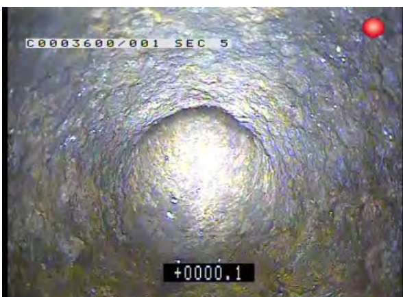
RWGX_0d509d9f-5890-4bb1-998b-04930288a1a0_20170824_1 131758_067.jpg, 00:04:04, 0.10m Line deviates up
