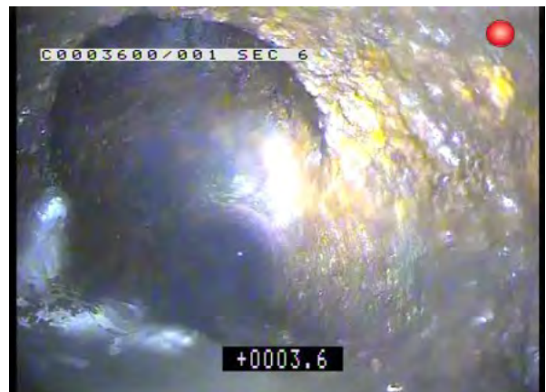
SW1X_a6e38308-1e08-4efb-853a-517ced4cdb53_20170824_132217_886.jpg, 00:00:29, 3.60m Junction at 12 o'clock, diameter: 100mm
