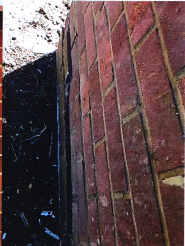
Lateral displacement of lower section of brickwork
