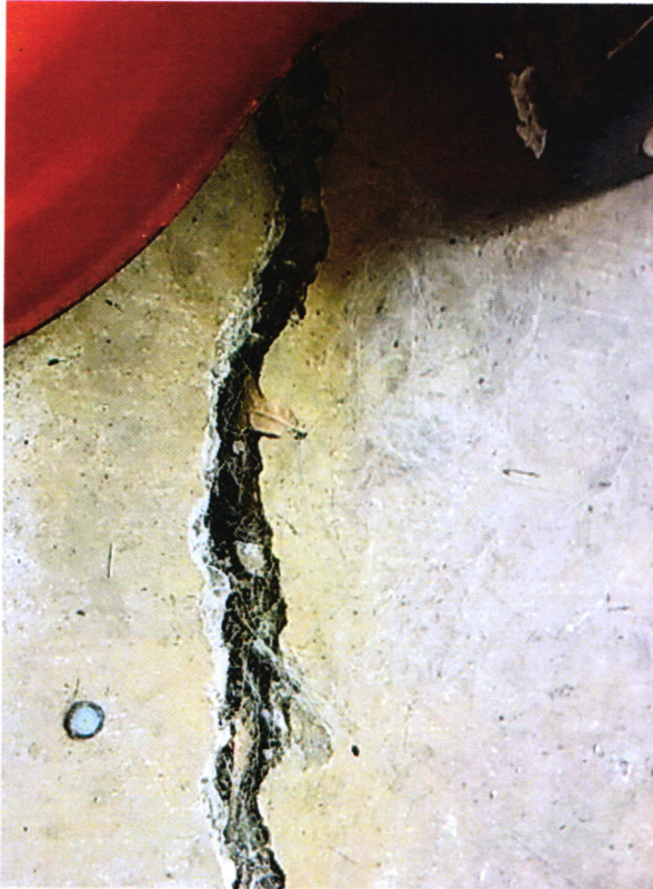
Fracturing to garage slab
