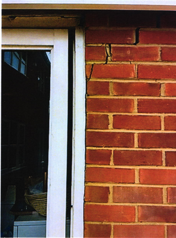
30mm gap between door and frame
