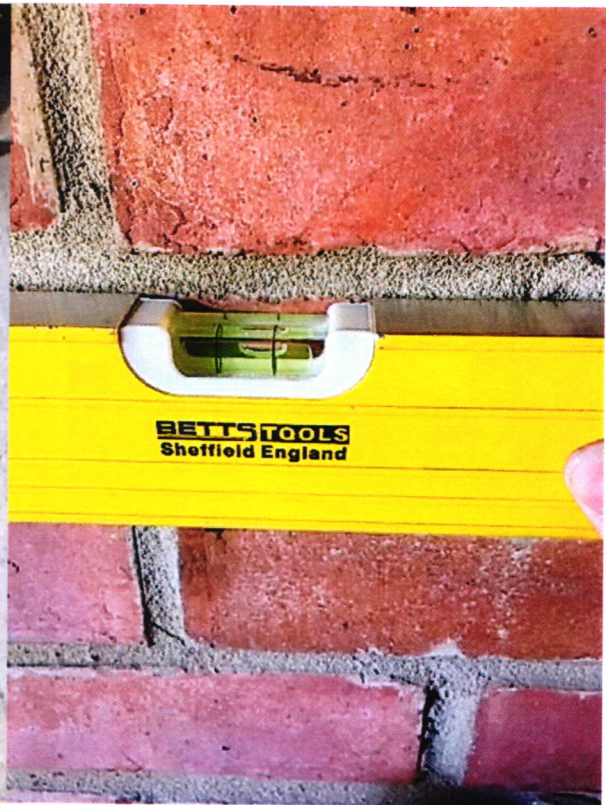
Distortion to brickwork
