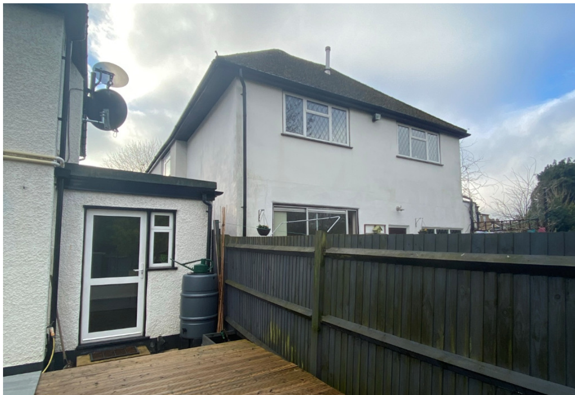
Above: Rear elevation of application property and neighbouring dwelling at No. 177.
