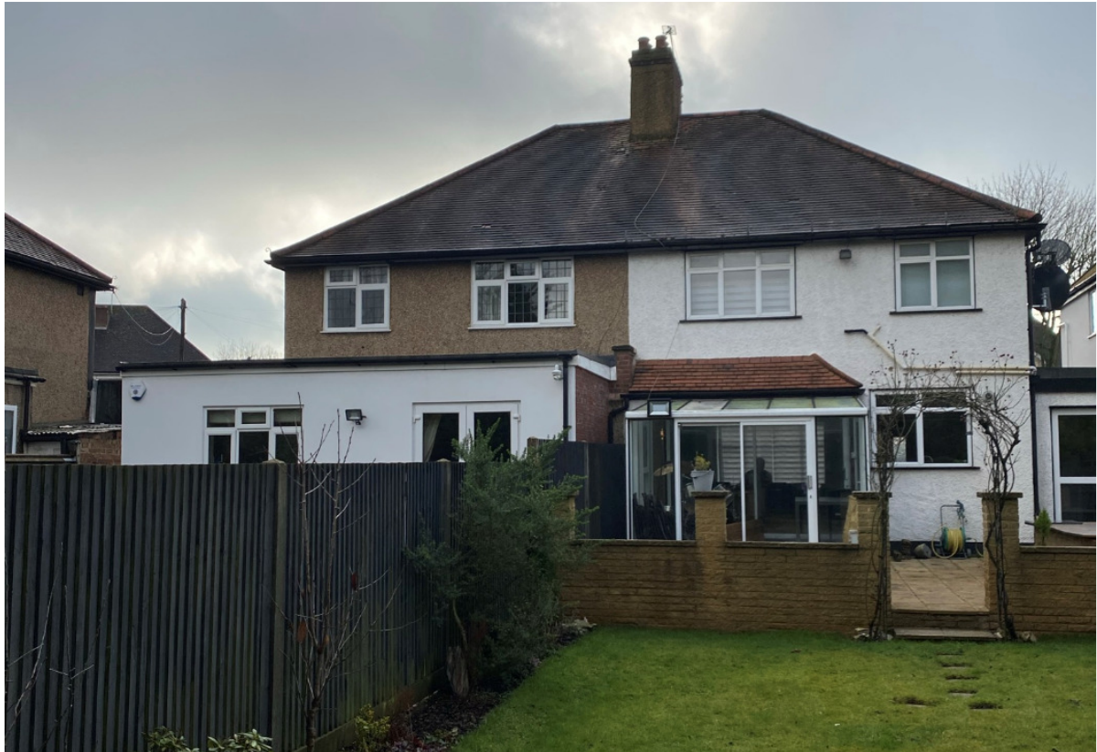
Above: Rear elevation of application property and neighbouring dwelling No. 181 – with single storey rear extension.
