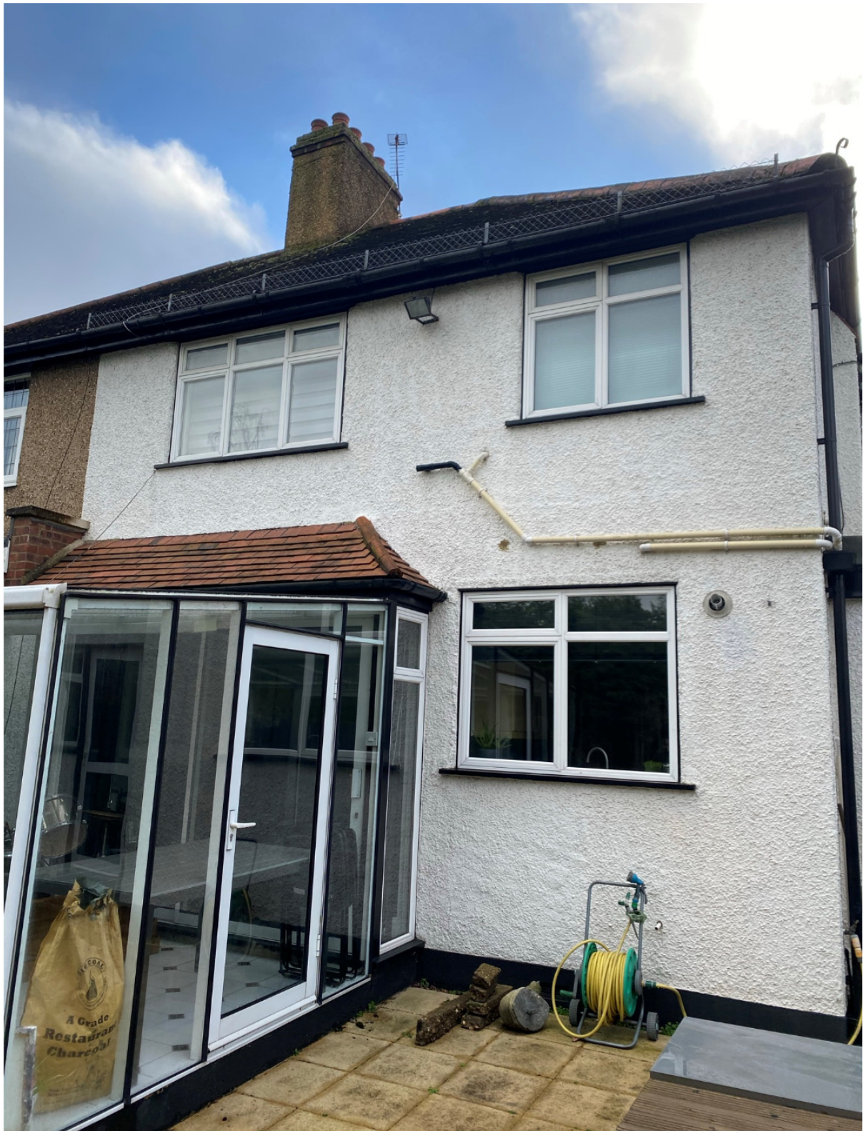
Above: Rear elevation of application property.
