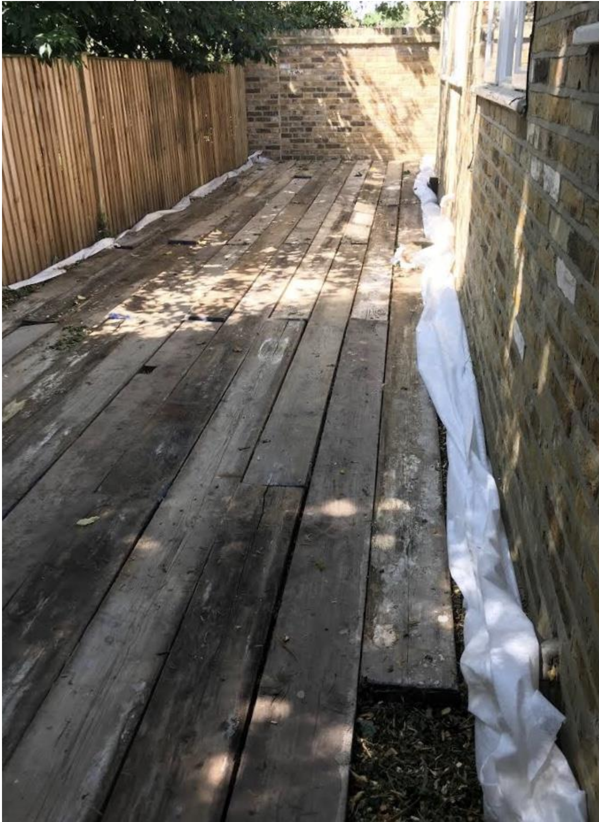
Photo 1. Scaffold boards placed on woodchip
