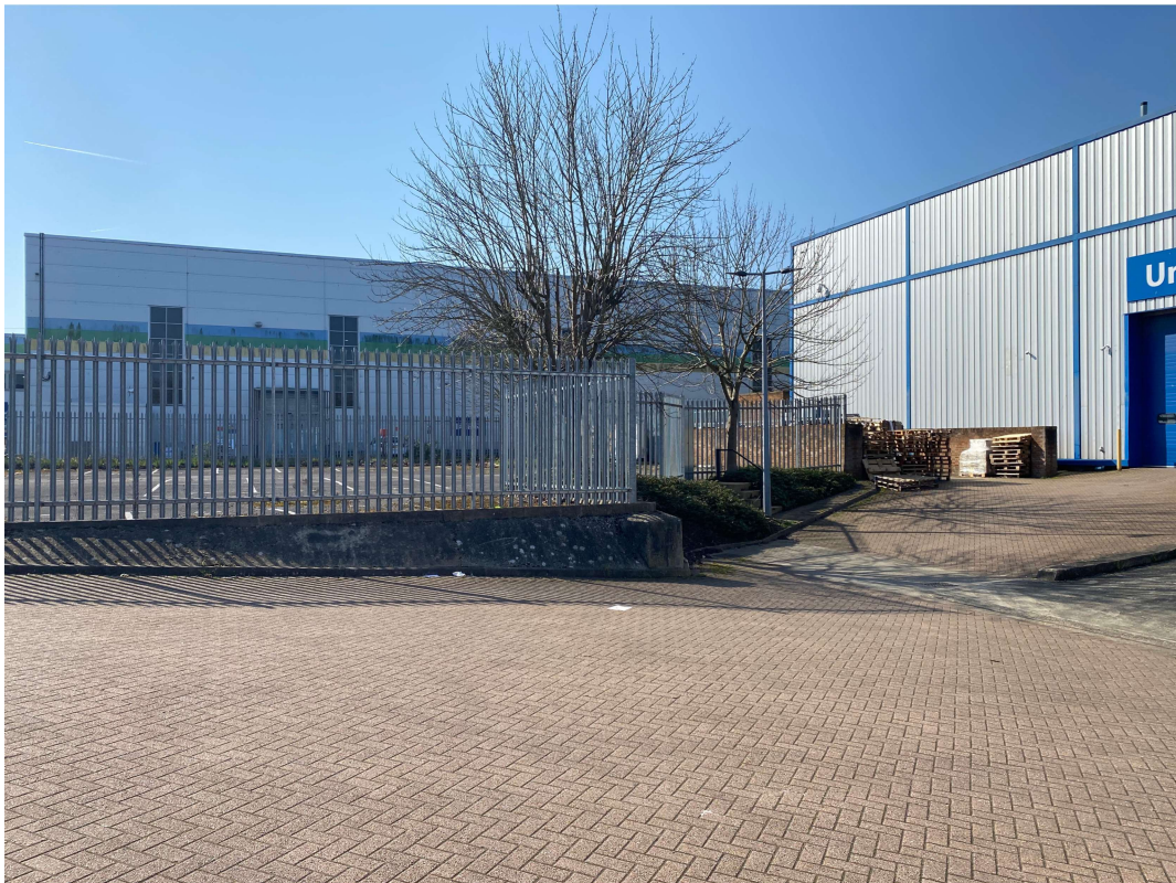
Car parking area to be removed to allow new loading bay doors to service the building
