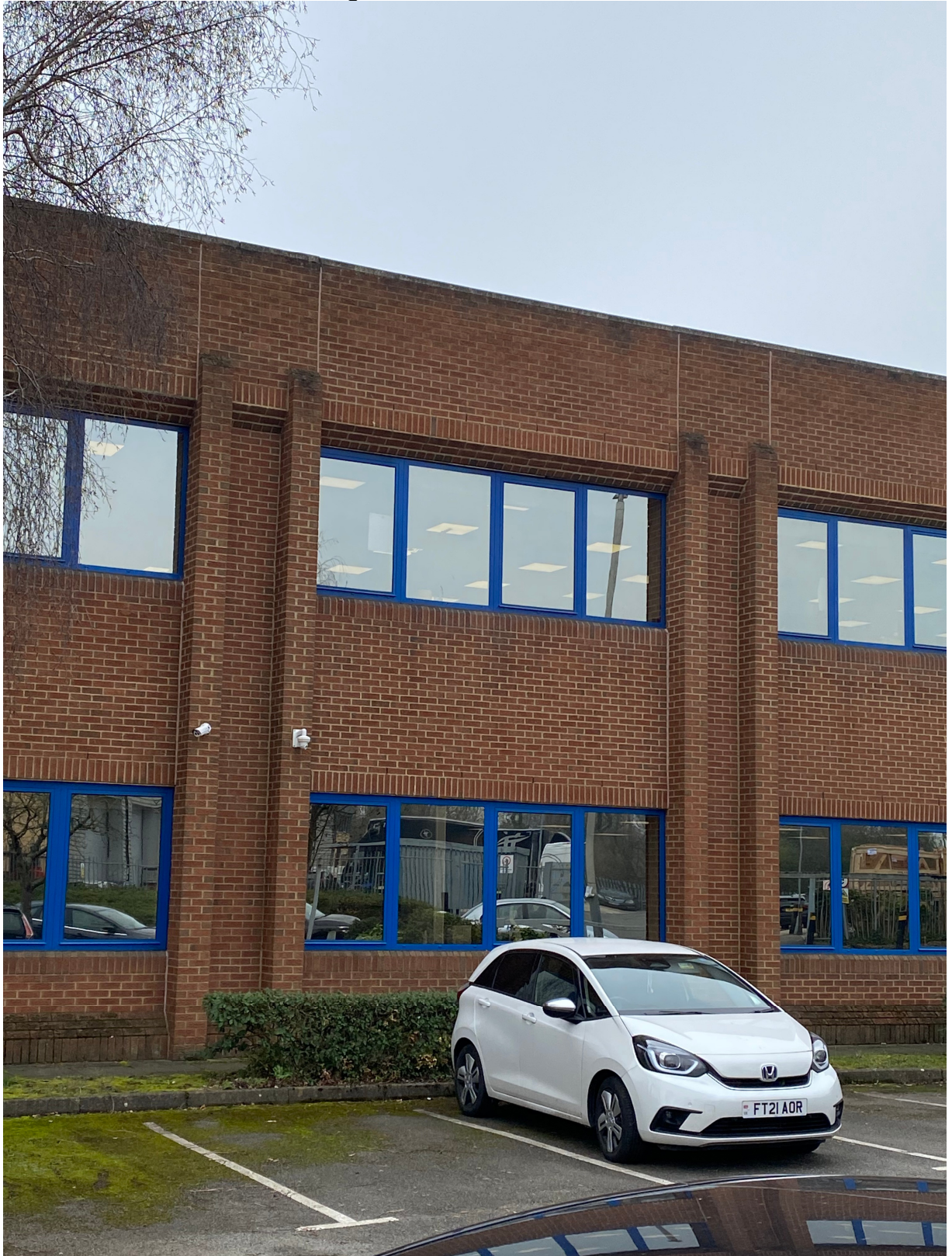
Typical office facade
