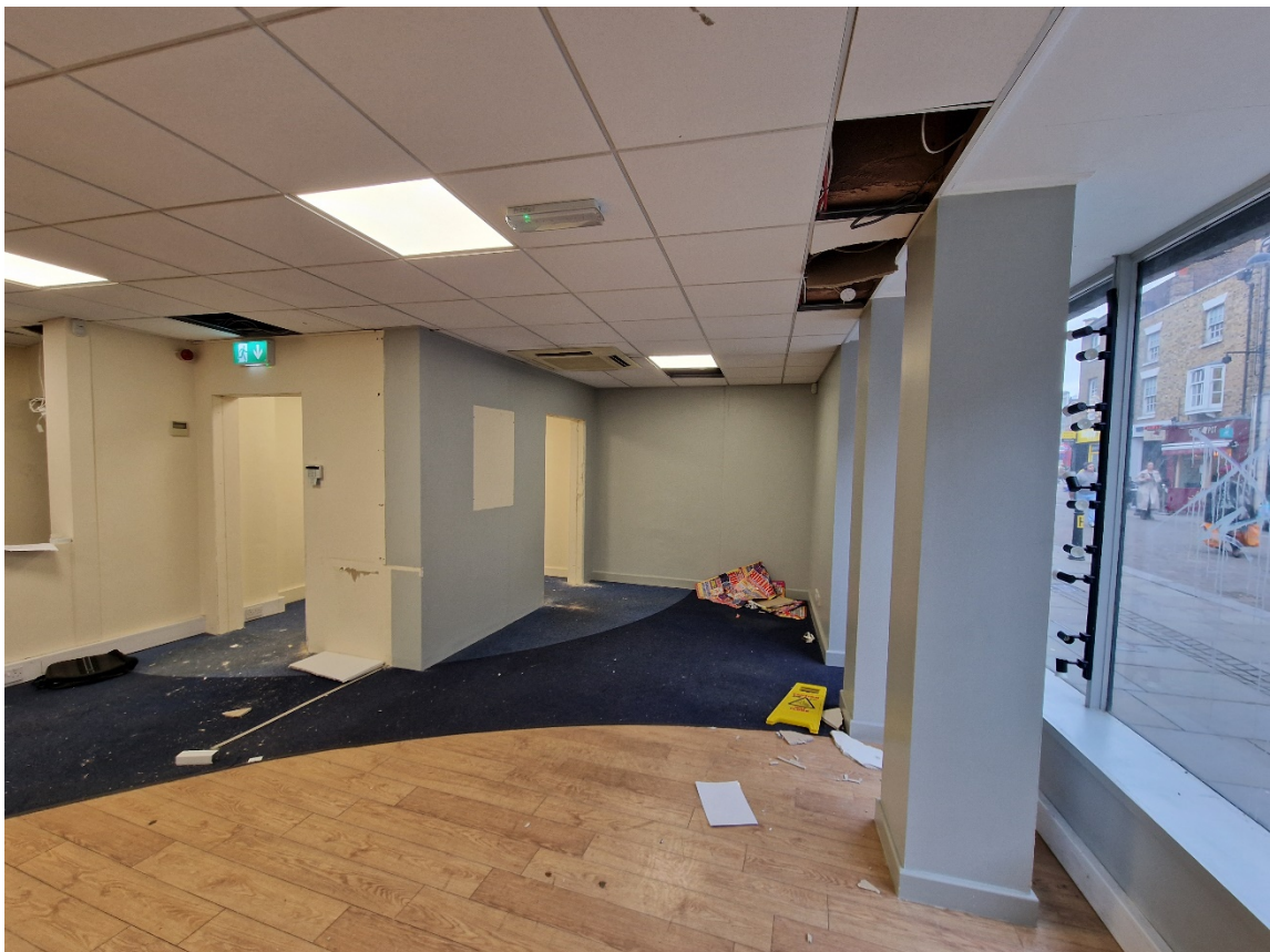
Internal walls only extend to suspended ceiling
