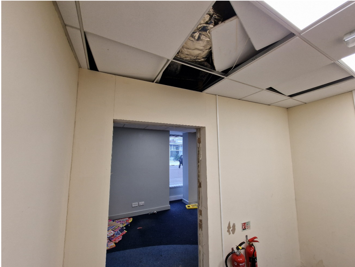
Internal walls only extend to suspended ceiling
