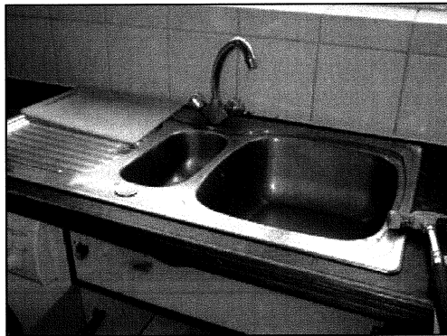
11/1/3B/31/PC5, Kitchen, Room ID G07, Sink Pad (No Asbestos Detected)
