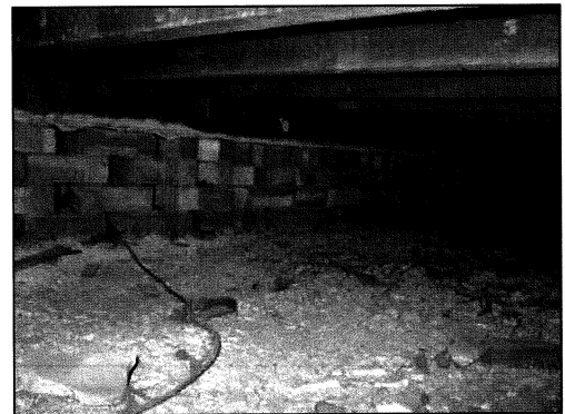
Bedroom, Room ID G04, Floor Intrusion (No Suspected Materials Seen)
