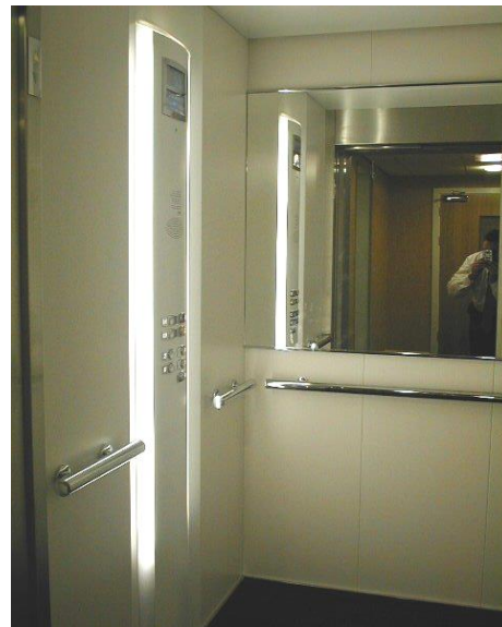
Typical Lift Interior View:
