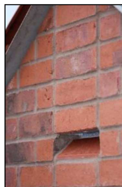
Figure 3: Habibat Bat Box faced with red brick, incorporated within wall at gable end.
