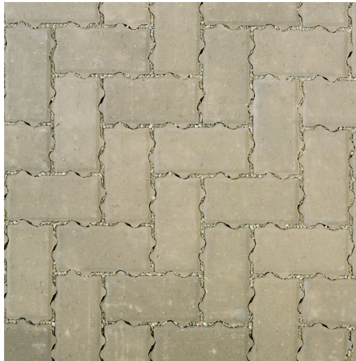
Car park surface - Brett Omega Flow Permeable Block
