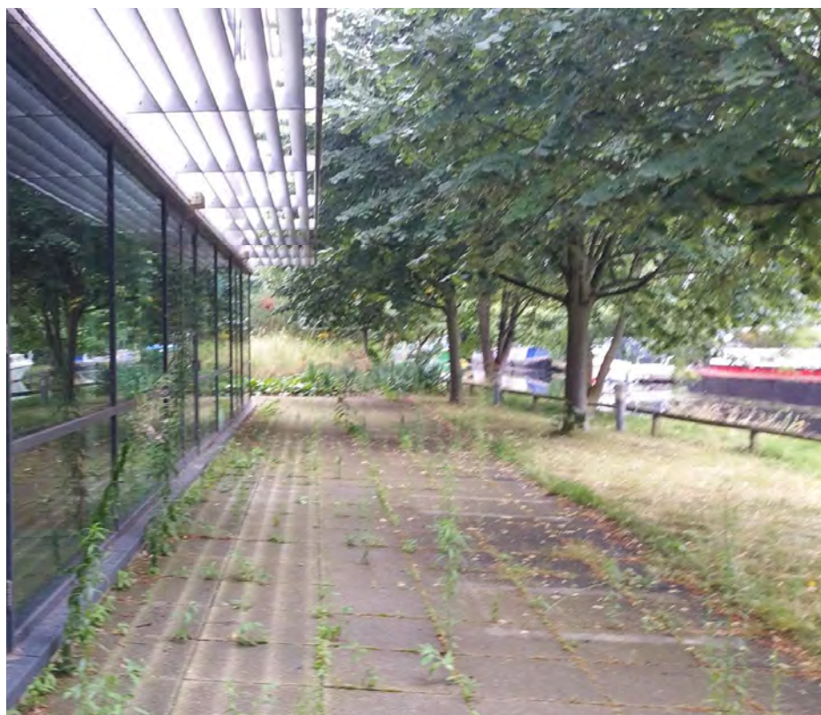
View South with two storey office building to left hand side and canal to right hand side
