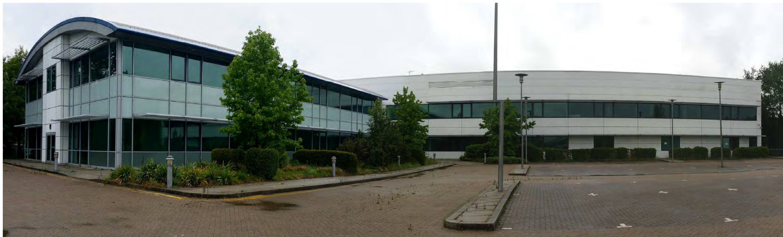
View of Car park and office annexe (left)
