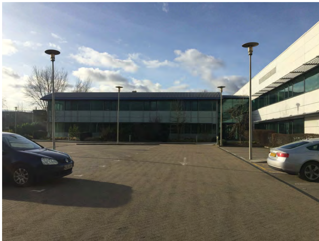
East elevation of office annexe and car park
