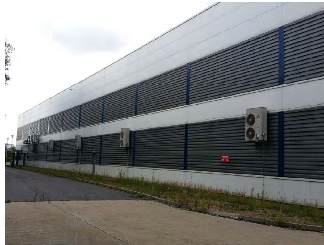
East elevation of warehouse
