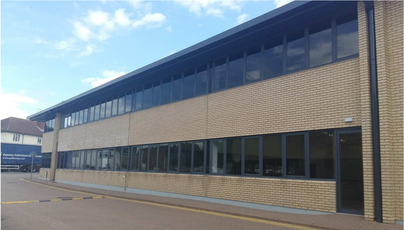
2. Existing building as viewed from outside.
