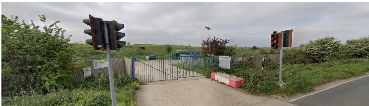
Photograph 2: Existing view from Harmondsworth Lane looking south into the former site entrance to Harmondsworth landfill.
