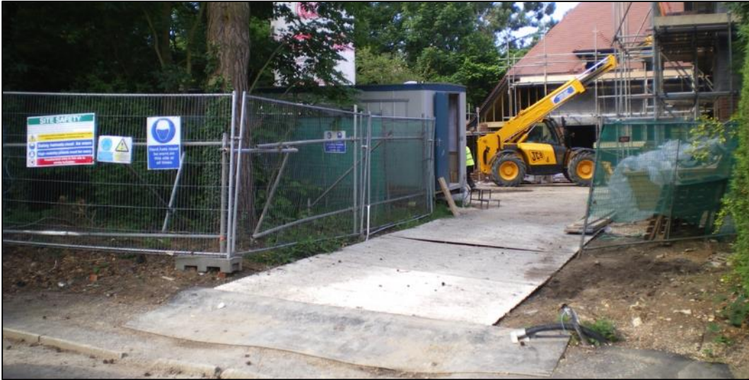
Vehicular ground protection trackway
