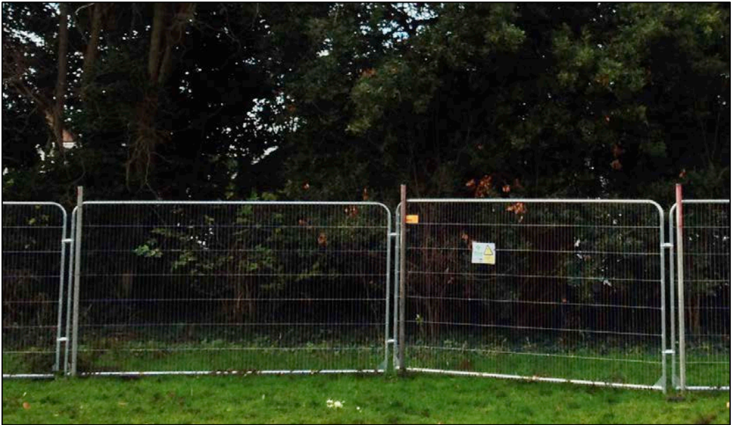
Weld-mesh panels on scaffold uprights
