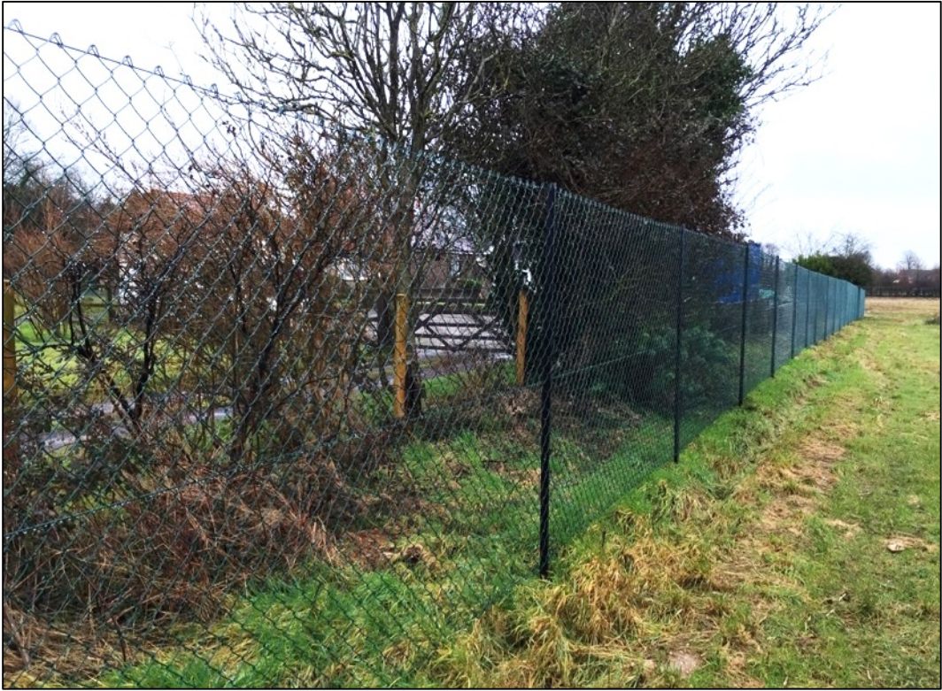
Chain-link on angle-iron uprights
