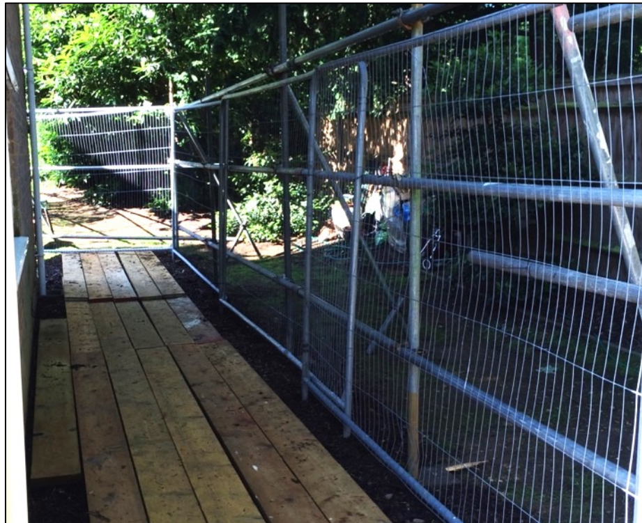
Scaffold board pedestrian ground protection
