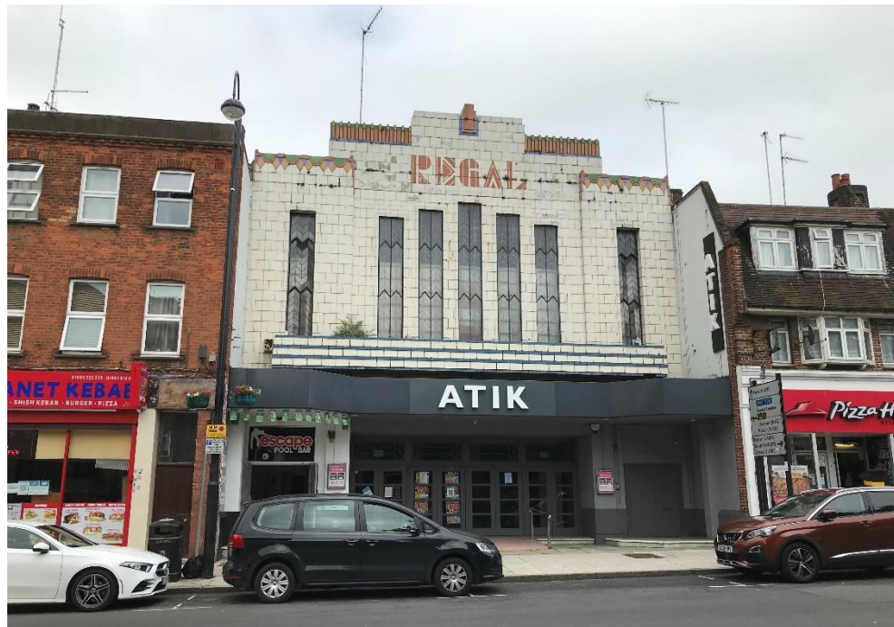
Figure 6: Main elevation of the GII* Discotheque Royle
