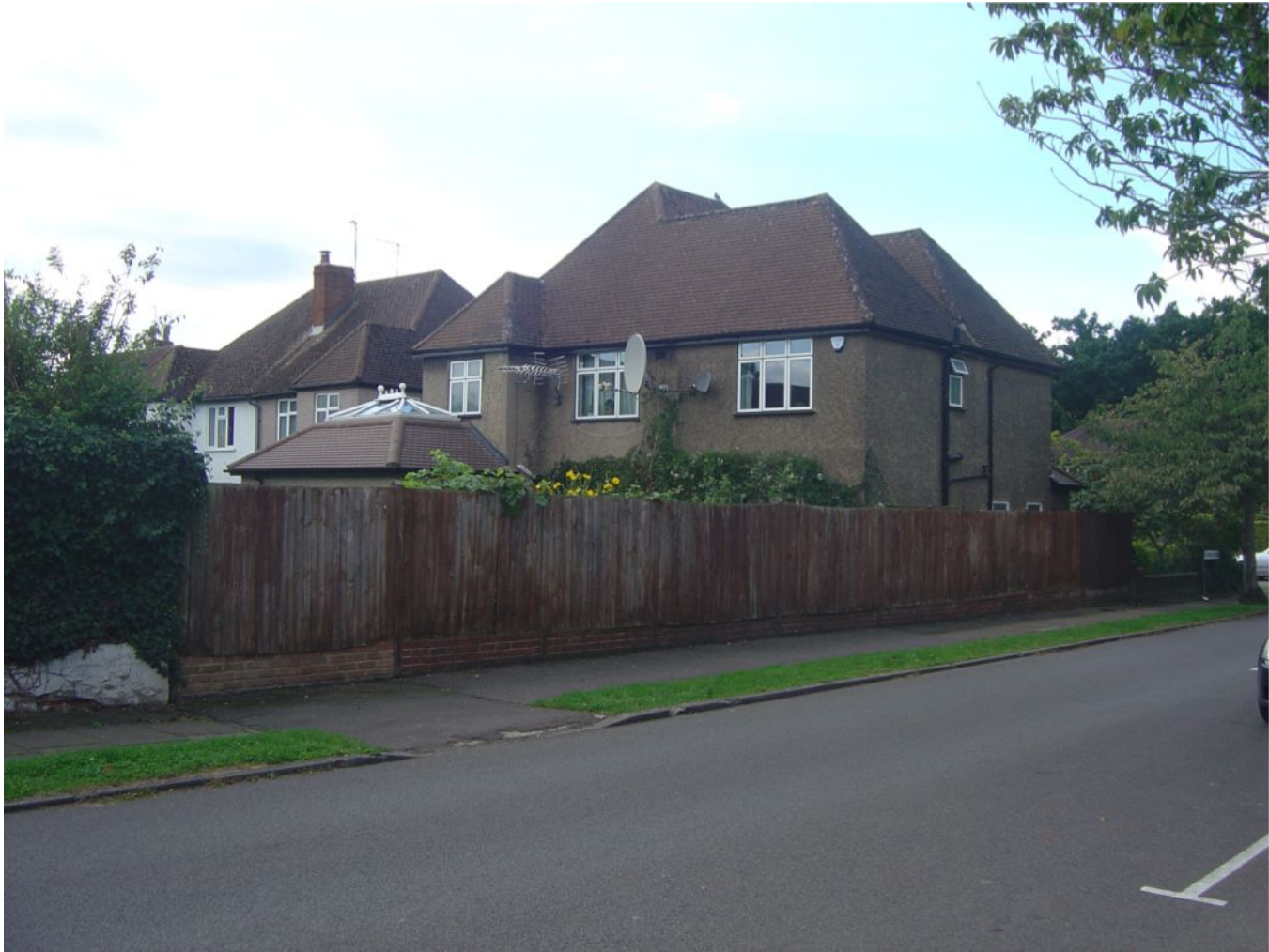
Existing photo from Almond Avenue
