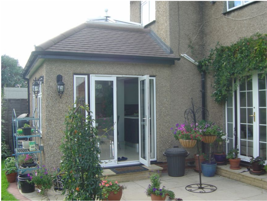
Existing rear extension to kitchen
