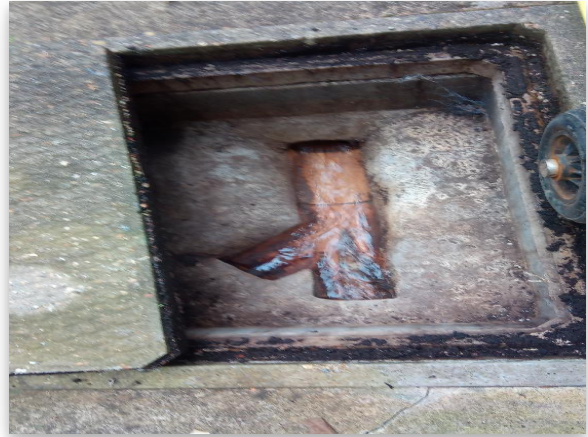
Fig 3.4: Manhole 3 (root ingress in chamber)
