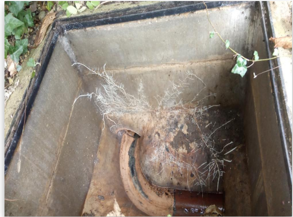
Fig 3.4: Manhole 3 (root ingress in chamber)
