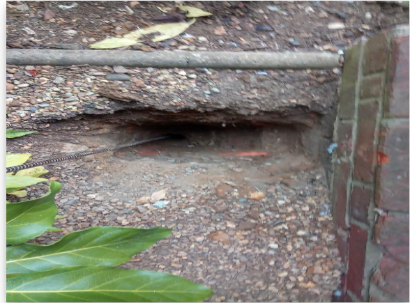
Fig 1.2: Trial Hole 1 Footing
