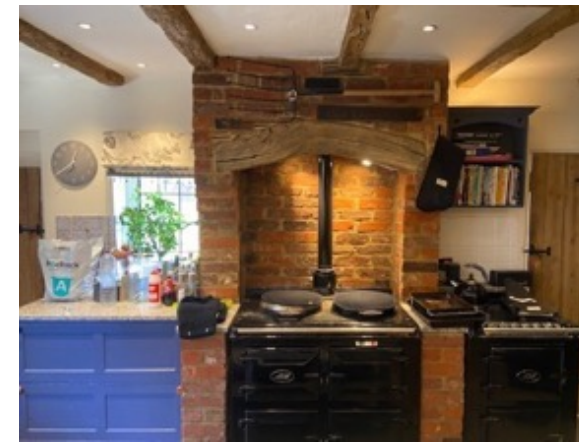
21. Proposed removal of non-original brick/ Aga surround
