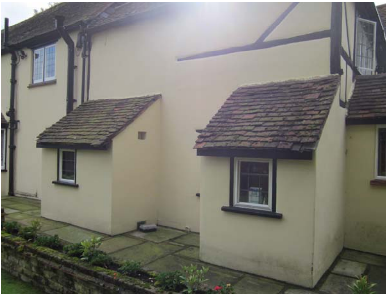
a. Area where the proposed two storey extension is to be located
