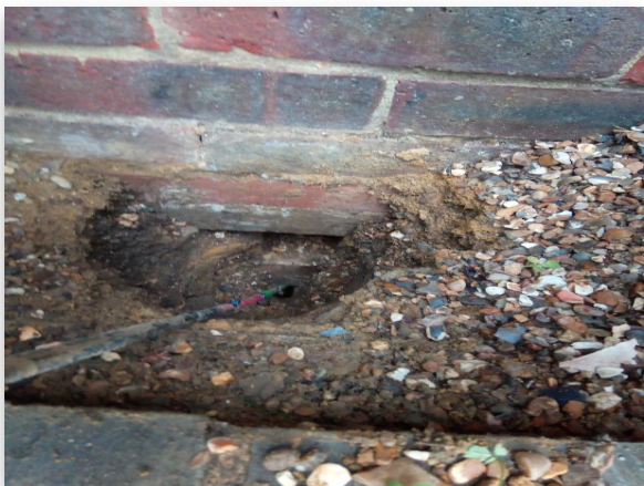
Fig 1.2: Trial Hole 1 Footing
