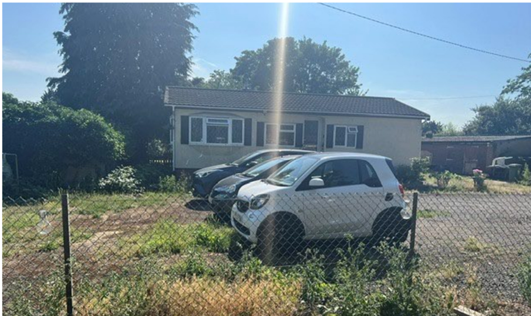
Ancillary office on land at Oakdene
