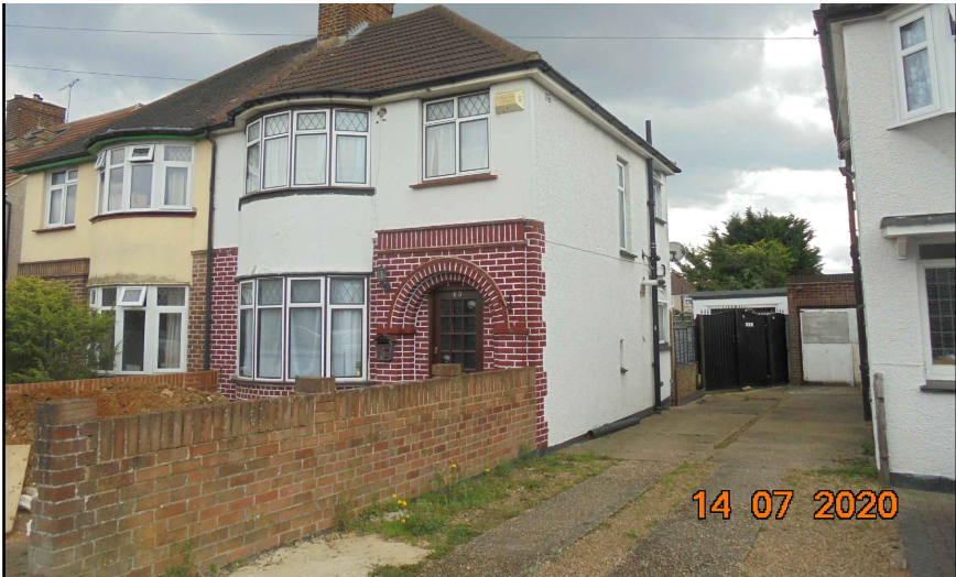
Existing Side View
