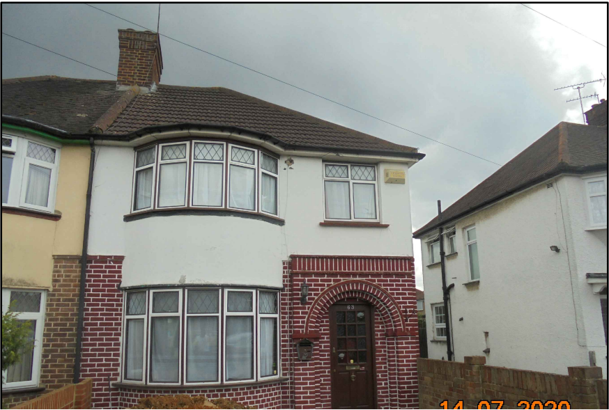
Existing Front View
