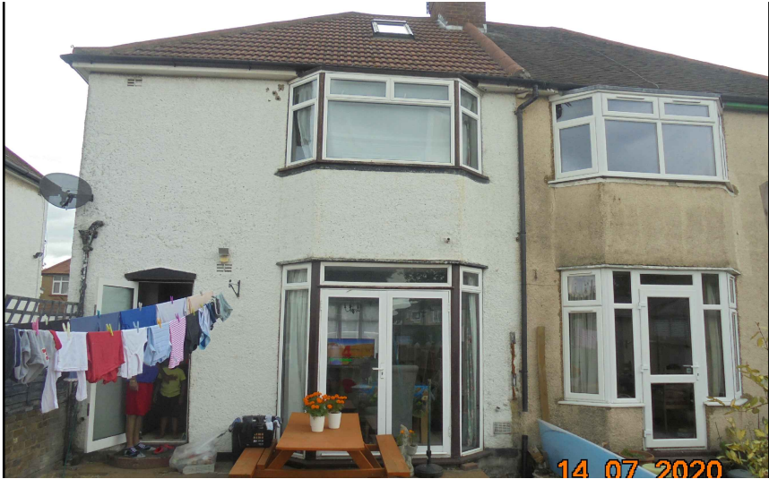
Existing Rear View
