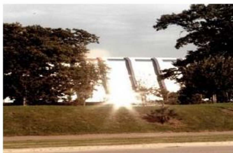
Solar glare on a sloping façade
