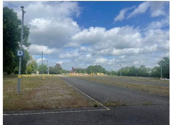
Figure 2.8: Car parking area viewed from the south-west corner of the site. Parking bays with an aggregate surface are overgrown with weeds and grass. Asphalt roads provide an accessway to the parking bays. Street lighting and CCTV facilitate the car park.
