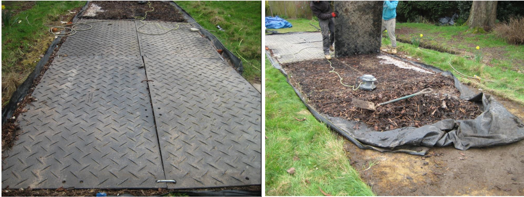
Fig 10 – Temporary ground protection is an effective way of allowing access through the RPA of retained trees. It must be installed prior to any on site activity and maintained for the duration of all works to be effective. Above left Tamla Trees project ground protection in place and above right being removed following the completion of site works. (Note: depending on the length of time it is in place it will adversely affect underlying grass ground cover which will need reseeded/ turfed accordingly)
