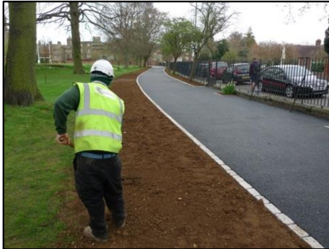
Fig 9 – All 'making good' topsoil will be BS3882 compliant and raked out by hand to no greater depth than 100mm
