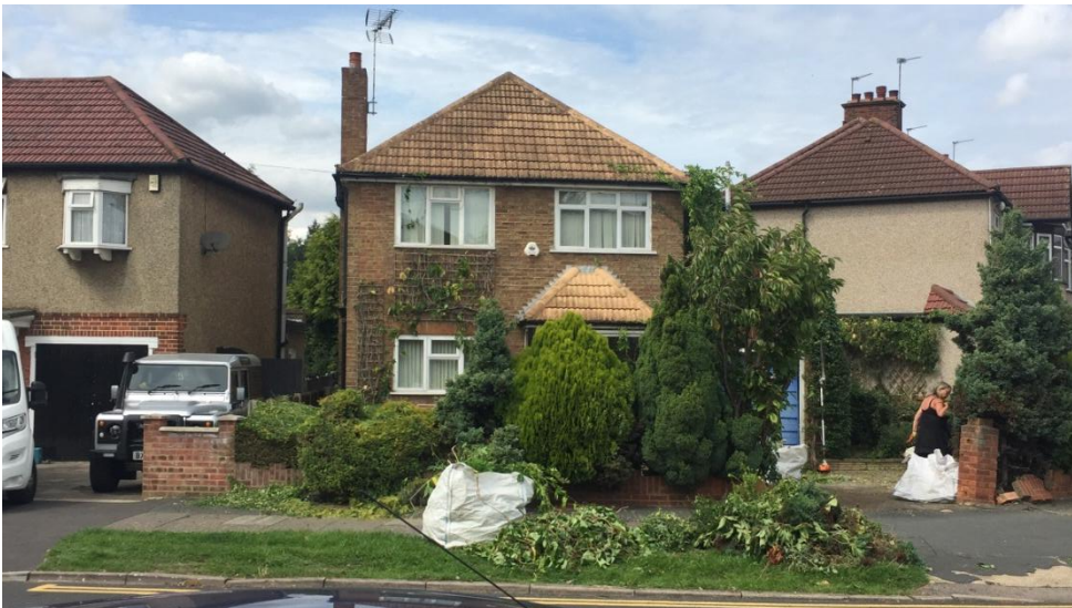
Figure 2: 7 Torrington Road; detached building on terraced street.
