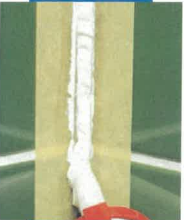
Application of Mapesil AC
