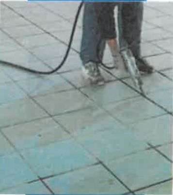
Sealing ceramic tile floor with Mapesil AC
