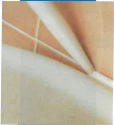
Sealing sanitary ware
