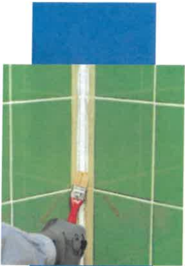
Smoothing the joint with soapy water and a small brush
