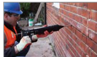
5. Insert a further bead of HeliBond over the exposed HeliBar, finishing 12mm from the face, and 'iron' firmly into the slot using the HeliBar Insertion Tool
