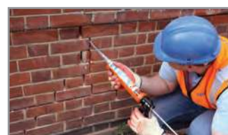
6. Re-point the mortar bed and make good the vertical crack with CrackBond TE3
