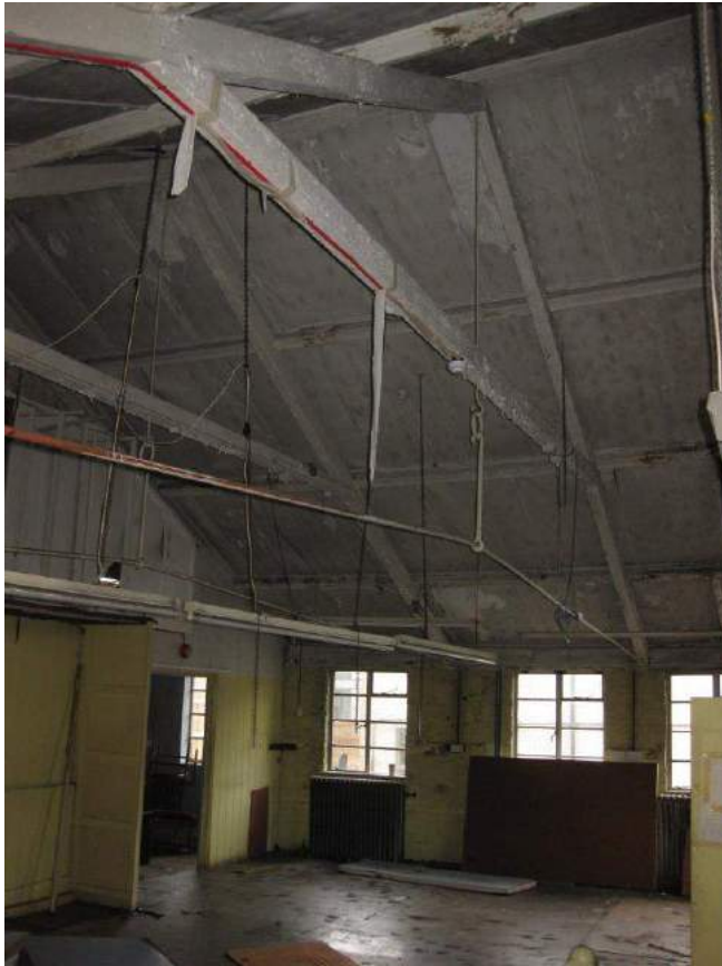
Figure 13: Tied timber trusses forming the roof structure to the rear of the building.
