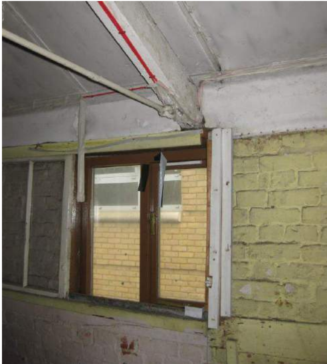
Figure 15: End of timber truss supported by a beam over an opening. Opening up works are required to determine the type and condition of the beam. The connection of the truss end to this beam is to be determined following opening works.
