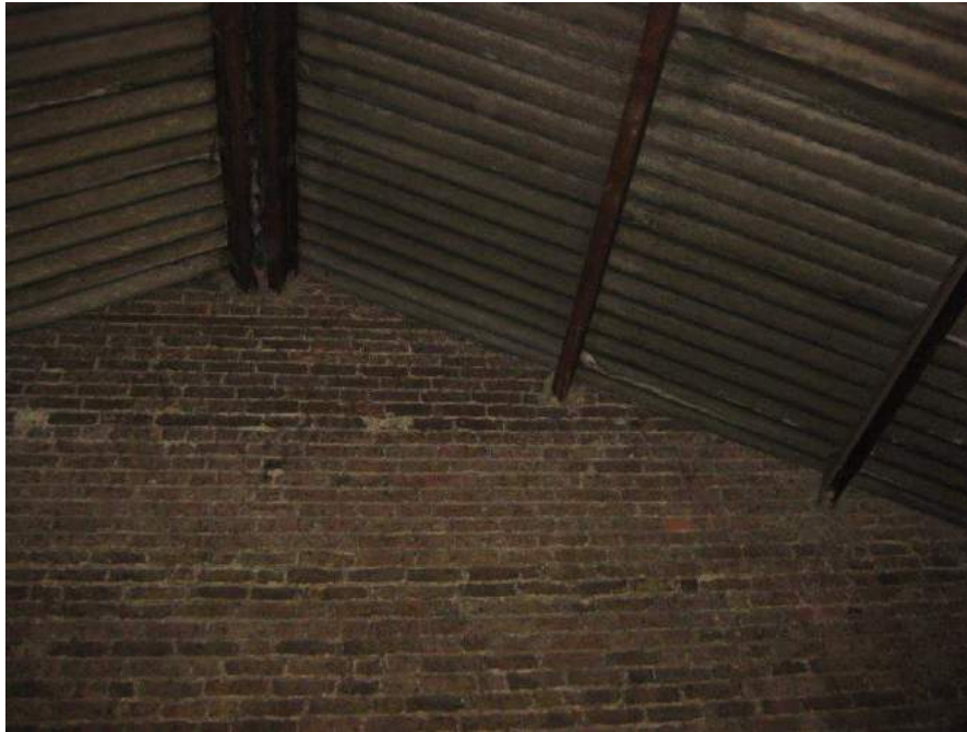
Figure 19: The rear wall of the fire station building at the interface with the 1960s warehouse. The warehouse roof purlins bear onto the fire station masonry wall.
