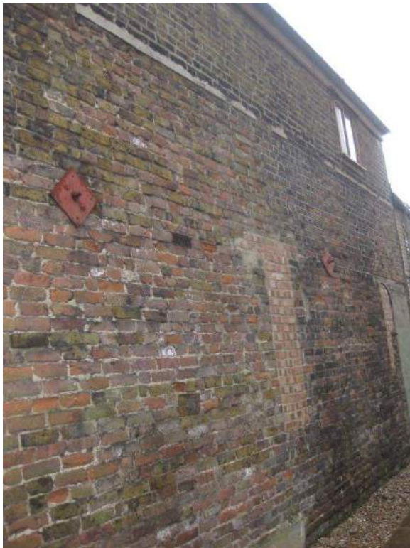
Figure 10: Side elevation next to Beaufort House. Historic infilling of openings present. Ends plates of tie rods visible.
