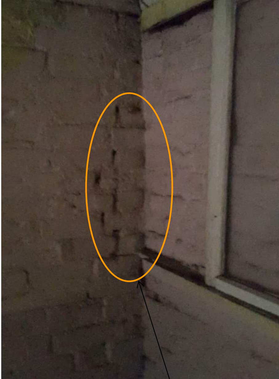
Internal view at south-east corner of building at first floor level
