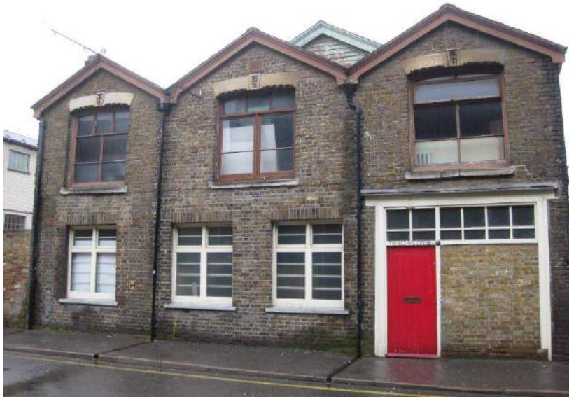
Figure 9: Front elevation. The ground floor elevation has been heavily modified since the building was first constructed.
