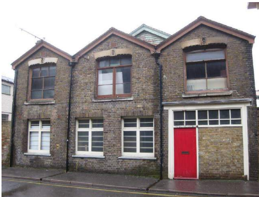
Figure 3: Current configuration of the fire station facade
