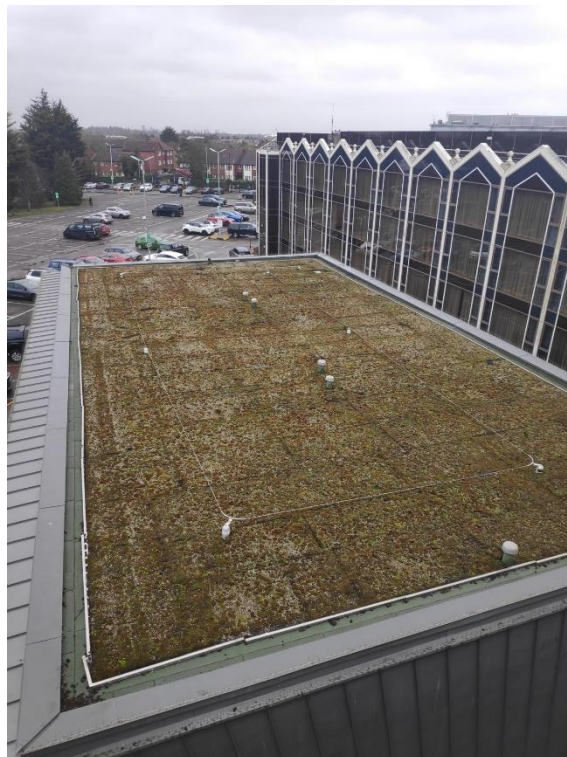
Photograph 4: Sedum roof to the extension
