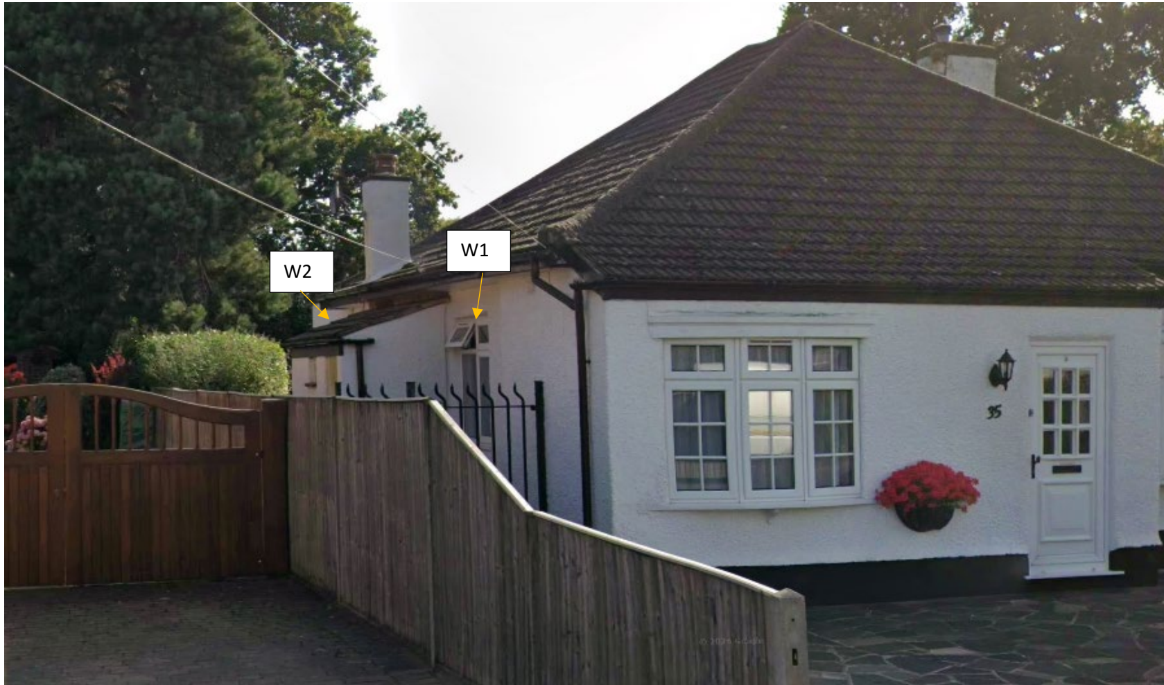
View of Side Elevation to 35 Parkfield Road
