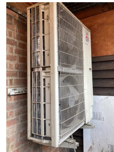
Existing air-conditioning condenser units that are to be relocated as part of the refurbishment
